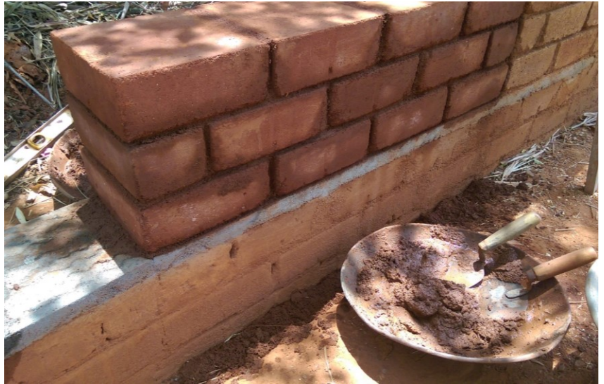
Compressed Stabilized Earth Blocks ( CSEBs )
