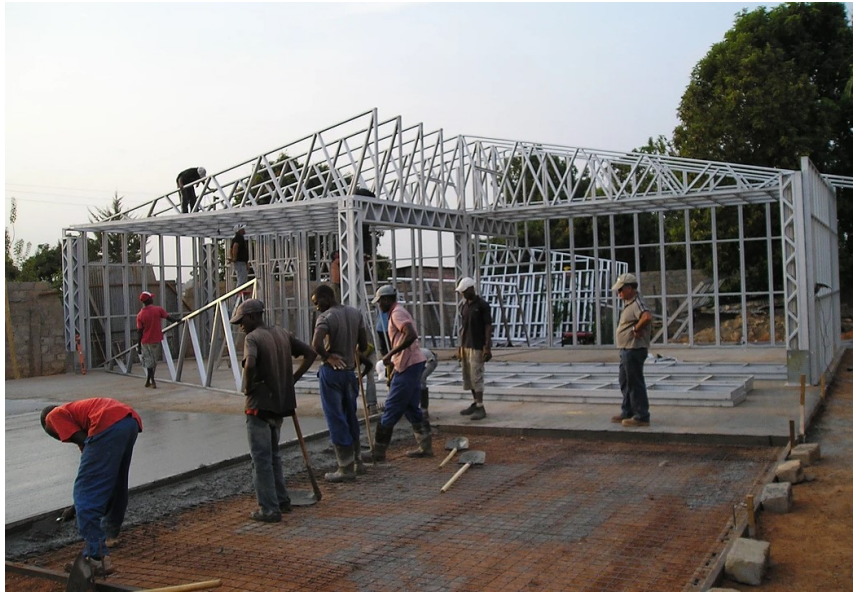
Steel Frame: Steel Home Company
